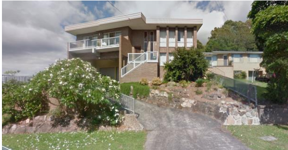
Figure 18: View of the existing residential dwelling at No. 12 Cosgrove Avenue looking east (Source: Google Streetview, 2013)
